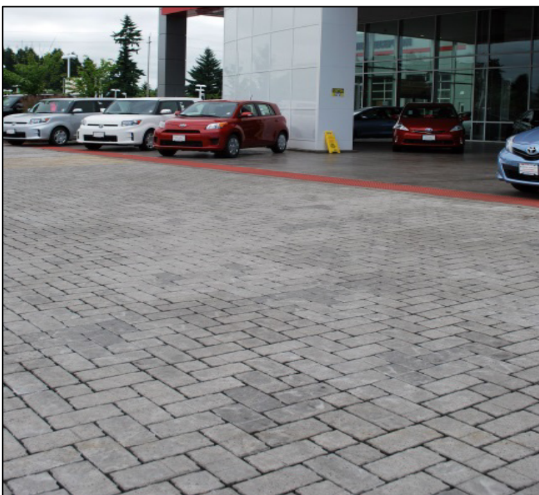
Figure 16: Permeable pavement application
