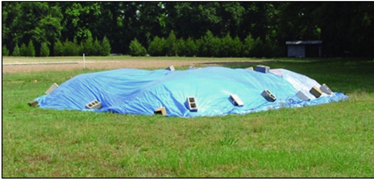
Figure 32: Covering a Stockpile
