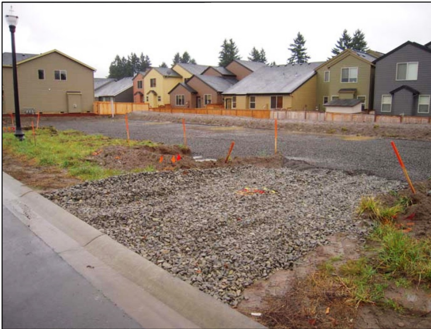
Figure 31: Small-scale Construction Entrance
