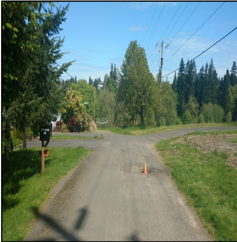
Before Construction 10 th Avenue / NE 154 th Avenue (View looking north)
