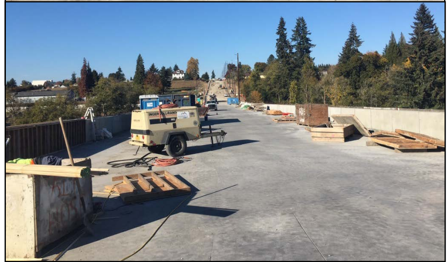
During Construction 10 th Avenue Bridge (View looking north)
