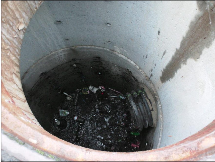
Drywell with Accumulated Trash
