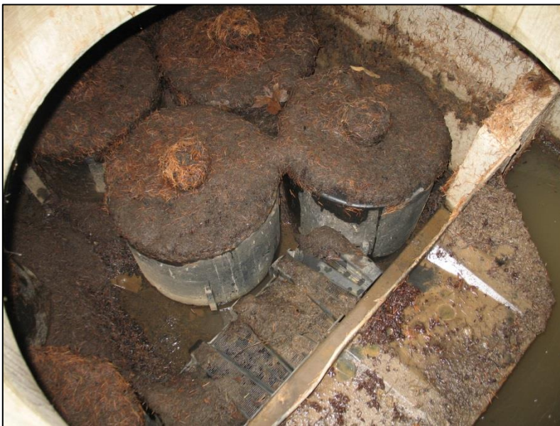
Media Cartridge Filter Vault with Accumulated Sediment
