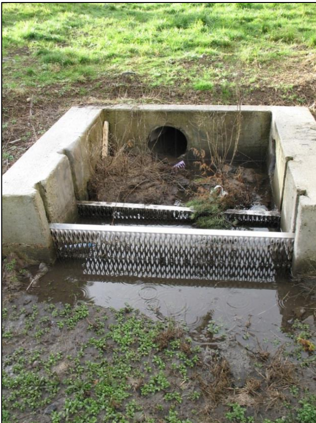
Sediment Trap with Accumulated Sediment
