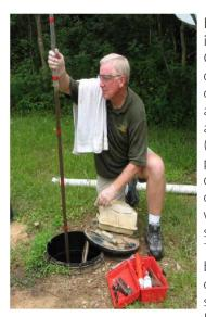
During the O & M inspection, the certified O & M specialist will determine if all the components of the OSS are properly working and/or need cleaning (e.g. pumps, filter, floats, pressure lines. drainfield, etc.) Also, the certified O&M specialist will verify the need for septic tank pumping. This will be determined by measuring the depth of septic sludge and scum in the septic tank. Inspection results are
