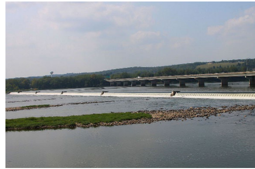
Adam T. Bower Memorial Dam in Pennsylvania
