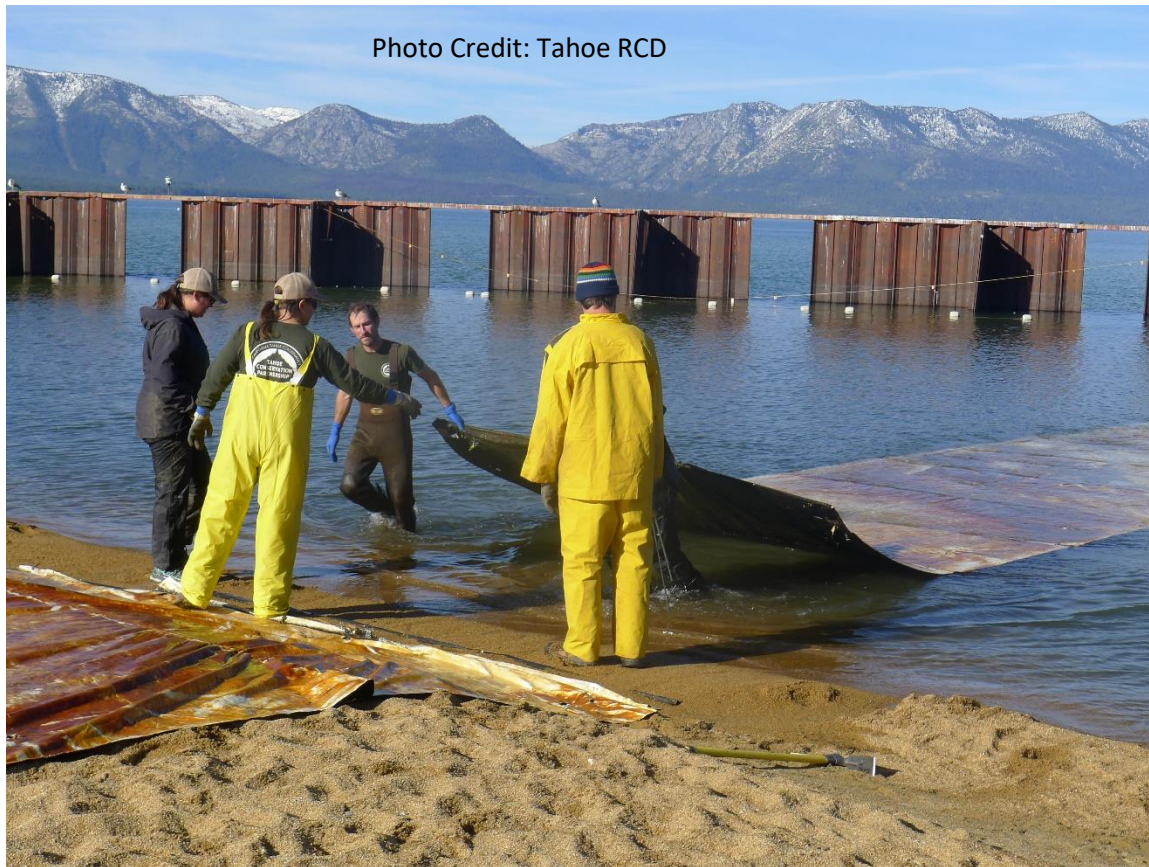
Figure 8. Workers using bottom barriers
