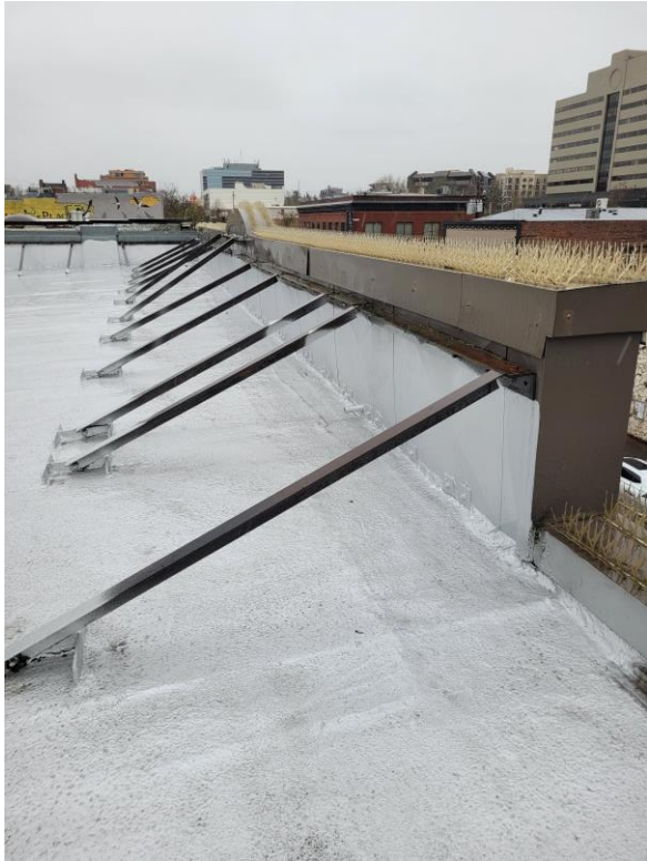
PARAPET BRACING
