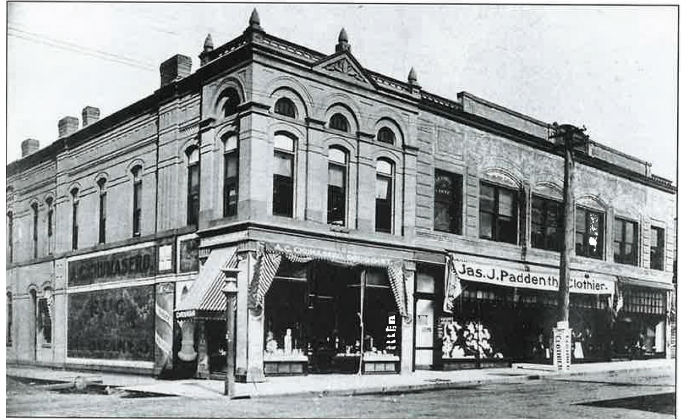
BUILDINGS 1&2: MAIN STREET SIDE
